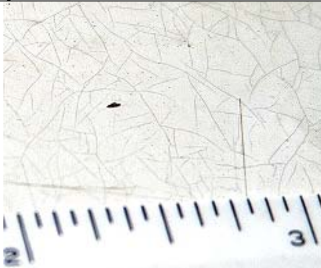
Figure 4 – Close-up enhanced photo of the micro-cracked/crazed powder coating on panel 01
