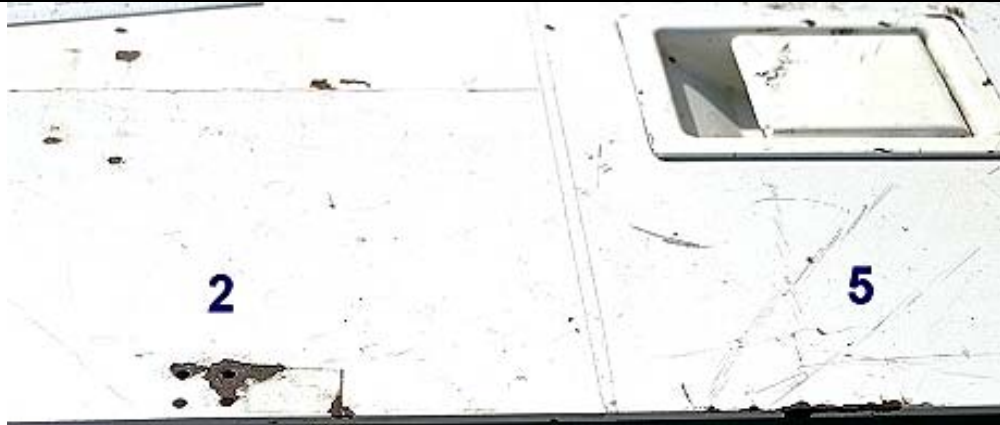
Figure 8 – Panel 01 - Damage noted on coating system 2 and 5
